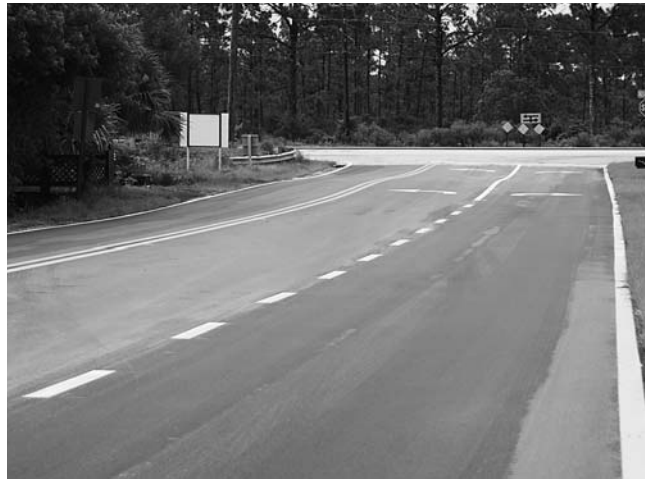
Asphalt overlay on Haynie Lane in Jupiter Farms
