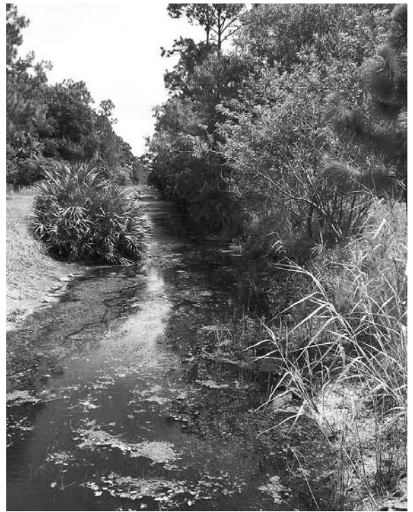
The District has over 60 miles of primary drainage canals
