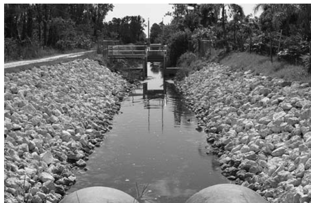
Restoration of canal banks funded by NRCS
