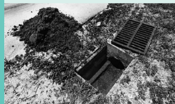
(Top) It is important to check underneath drainage grates for the accumulation of sediment, trash or debris. Pipe openings should be completely visible and free of any obstructions. (Center) It is always easier and less costly to remove any trash or build-up at this point – BEFORE it is carried further into the underground piping system. (Bottom) The removal of excess sediment will allow the structure to operate at its peak efficiency. Remember to properly dispose of the excess material and securely replace the drainage grates.
