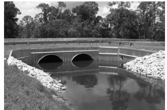
New culverts at Canal 2 and Jupiter Farms Road funded by NRCS
