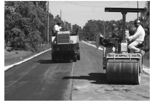
Road paving in Palm Beach Country Estates
