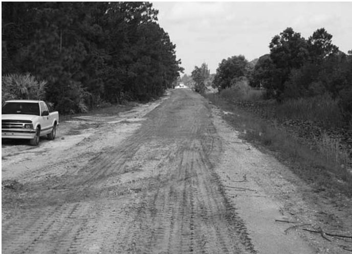
Palm Beach Country Estates levee restoration
