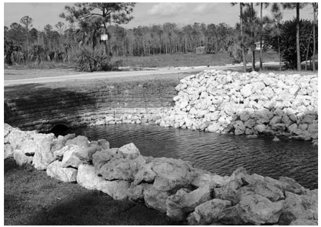
Riprap installation on a canal in Palm Beach Country Estates
