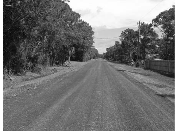
OGEM application on 80th Drive N in Palm Beach Country Estates
