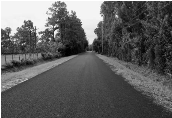
Rocky Pines OGEM-surfaced roadway
