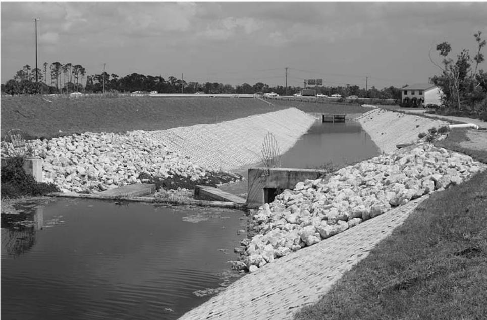
*The SR706 Outfall Canal project features concrete block mats and rip-rap that stabilize canal banks*
