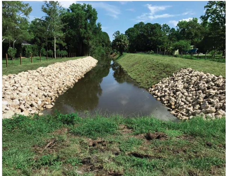
South Indian River Water Control District - Canal 3
