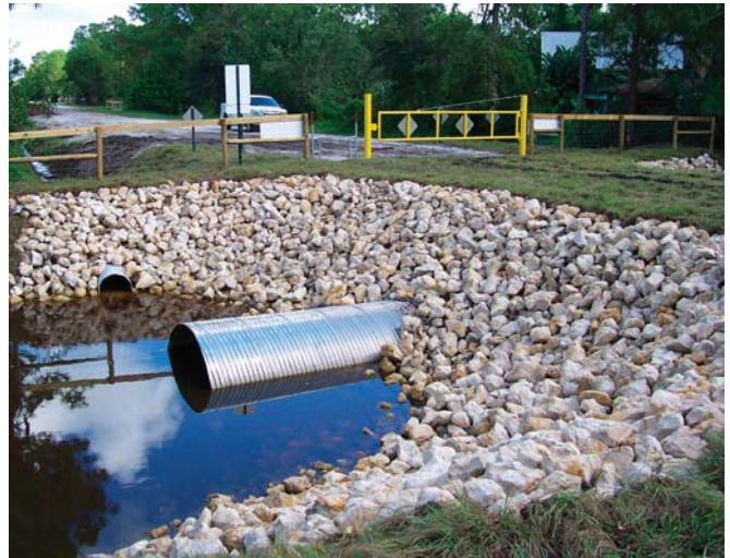
Culvert installation at Canal 7 and Alexander Run
